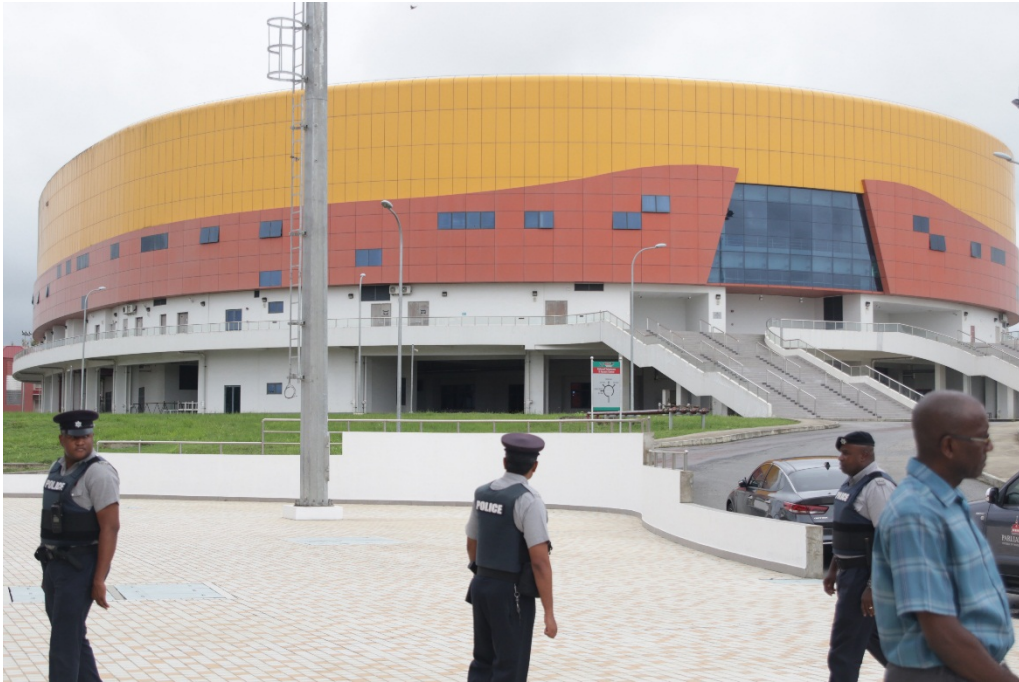
FIGURE 3 VIEW OF VELODROME FROM THE OUTSIDE
