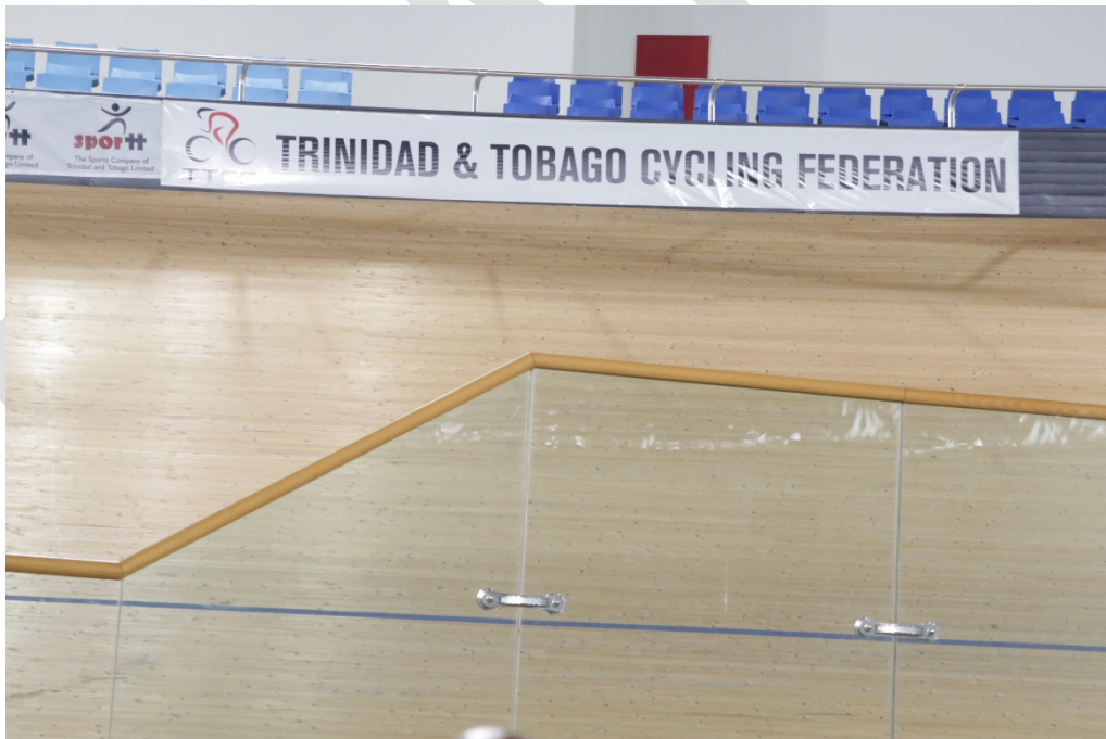
FIGURE 16 CLOSE-UP OF TRACK AT VELODROME
