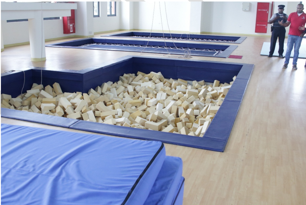
FIGURE 6 DEPLETED FOAM PIT AT DRY DIVING AREA, NATIONAL AQUATIC CENTRE
