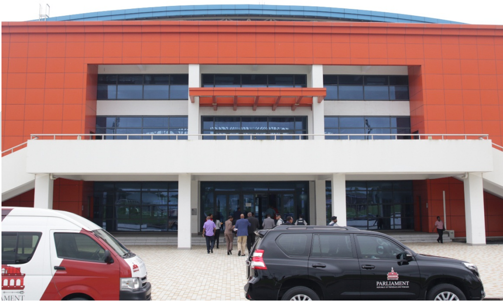
FIGURE 4 VIEW OF THE NATIONAL AQUATIC CENTRE FROM THE OUTSIDE
