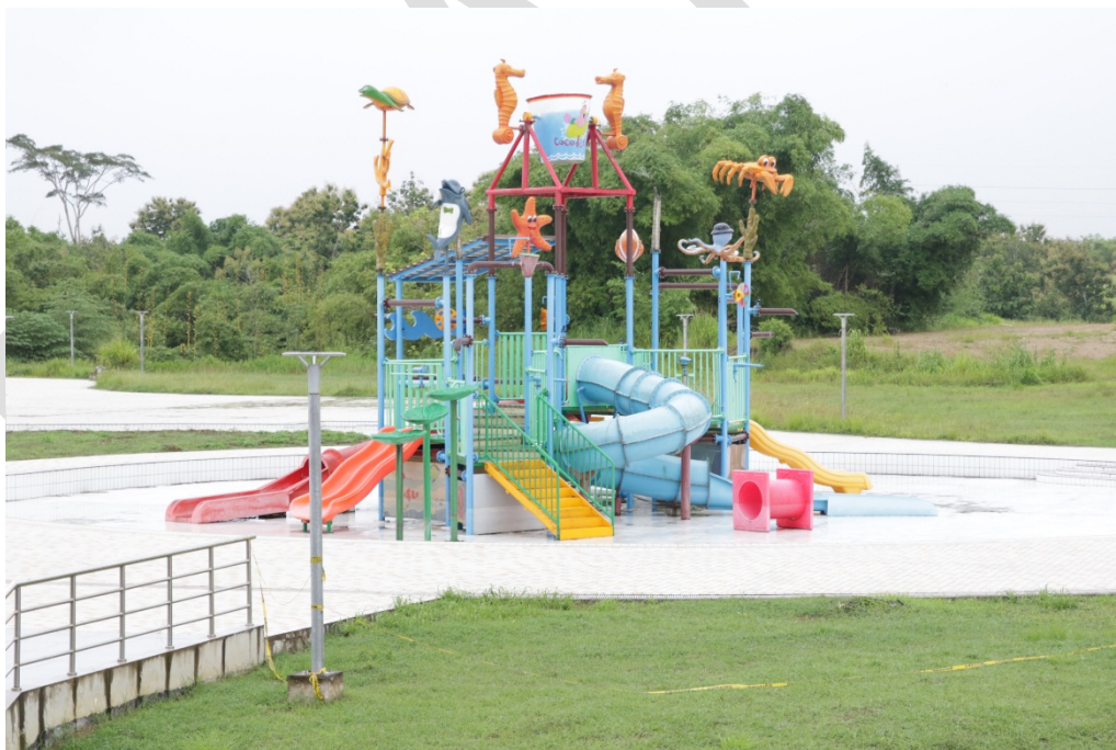
FIGURE 12 PLAY PARK DRAINED OF WATER TO VIEW DAMAGED AREAS
