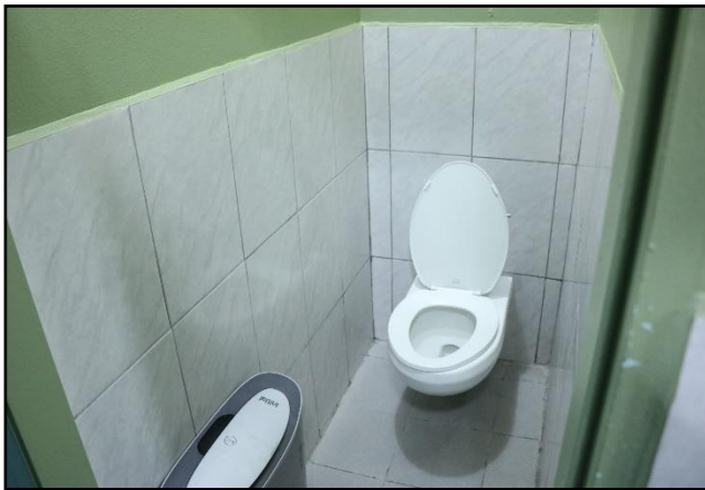
Figure 20: Toilet in the female dormitory
